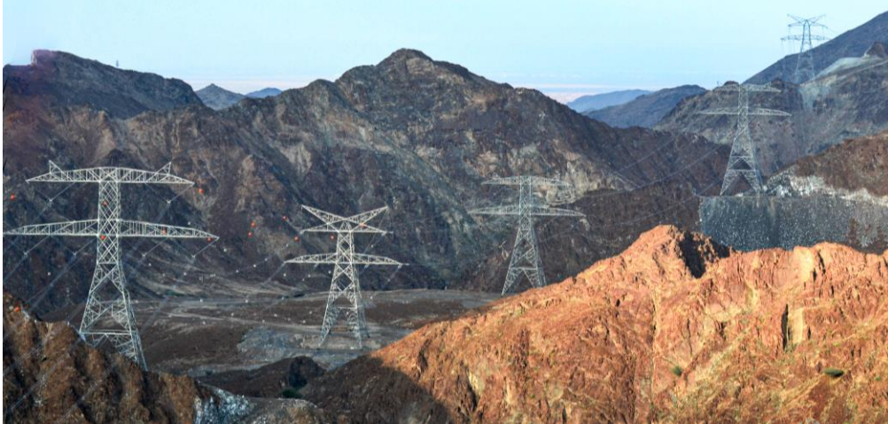
400 kV IBRI-New Rustaq O/H Transmission Line, Oman
