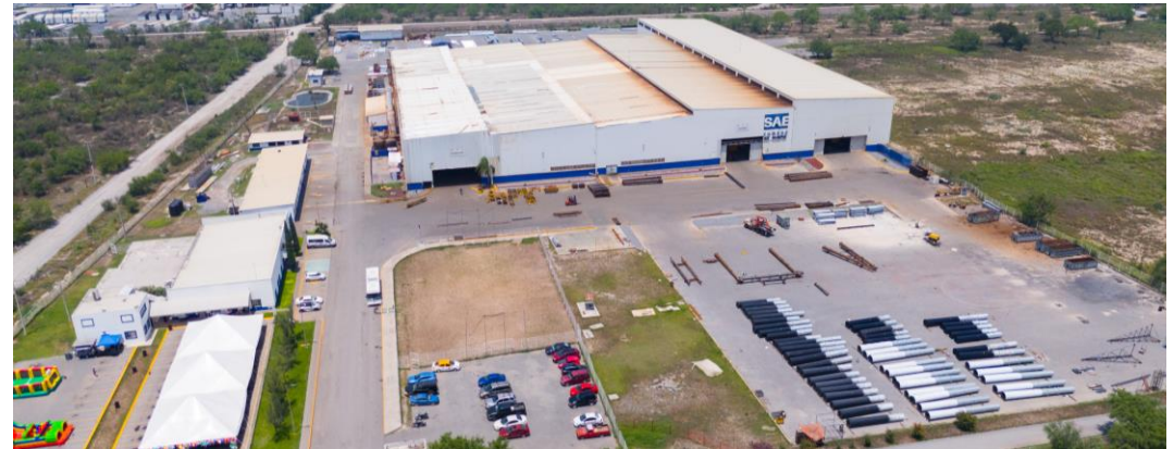
Tower Manufacturing Facility, Mexico
