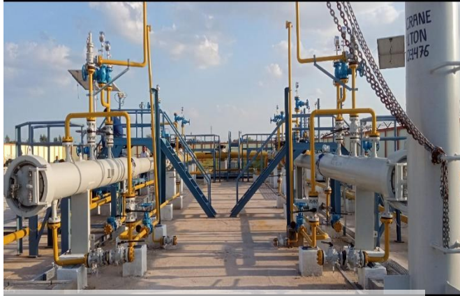
Station Piping Works at Sultanpur-Jhajjar Pipeline Project
