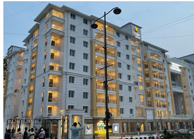
Construction of luxury residential project in Goa
